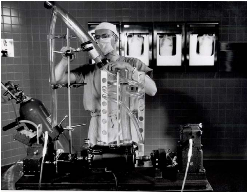
University of Minnesota's bubble oxygenator cost $15 and was easy to use. Richard DeWall is shown here with his model in 1955. University of Minnesota, Atlas of Human Cardiac Anatomy , https://www.vhlab.umn.edu/atlas/umn-cv-history/1951-56.shtml , accessed Jan. 16, 2024.
